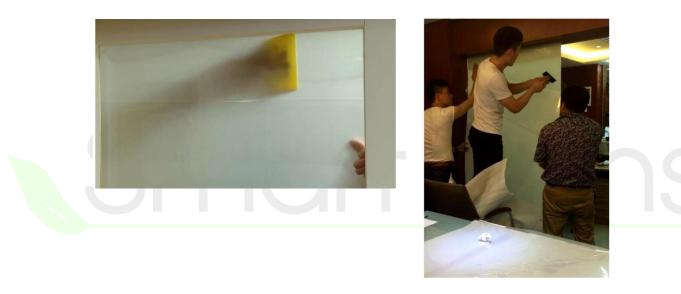
**Step 2.7:** Repeat the process (starting with step 2.5) until the installation is free of any air bubbles. Step 2.8 (below) should be paid close attention to, should air bubbles be trapped on the edges of the FILM.
